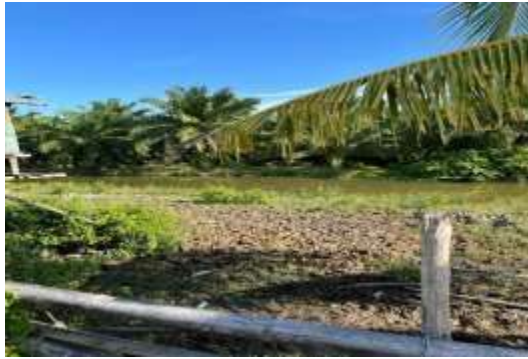
Fig. 2. Inland flooding due to severe seepage through the embankment.
