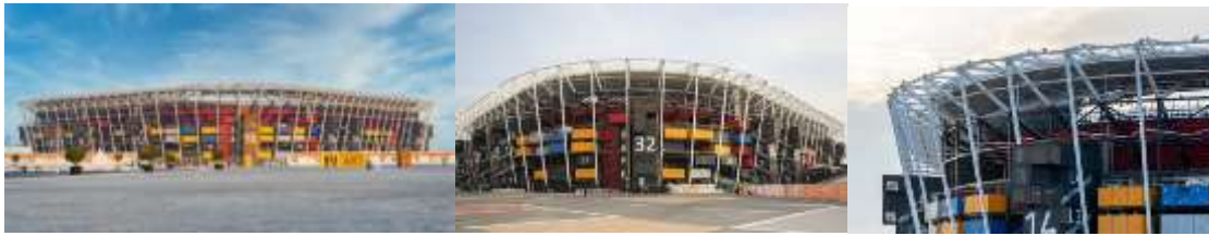
Figure 2. Container used as stadium, Qatar (Archdaily, 2022)
