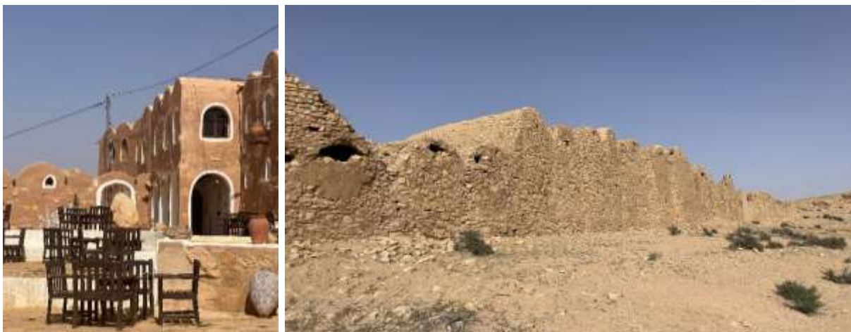
Figure 4: Ksar Ouled Debbab: The contrast between reused and abandoned site
