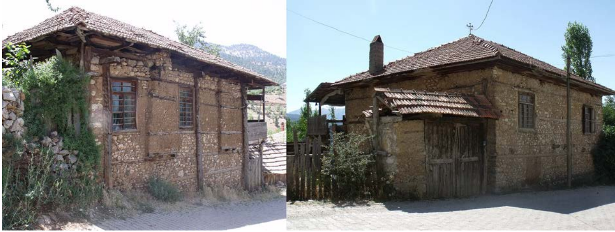
Figure 4. Traditional houses back facade with outer sofa (by author).
