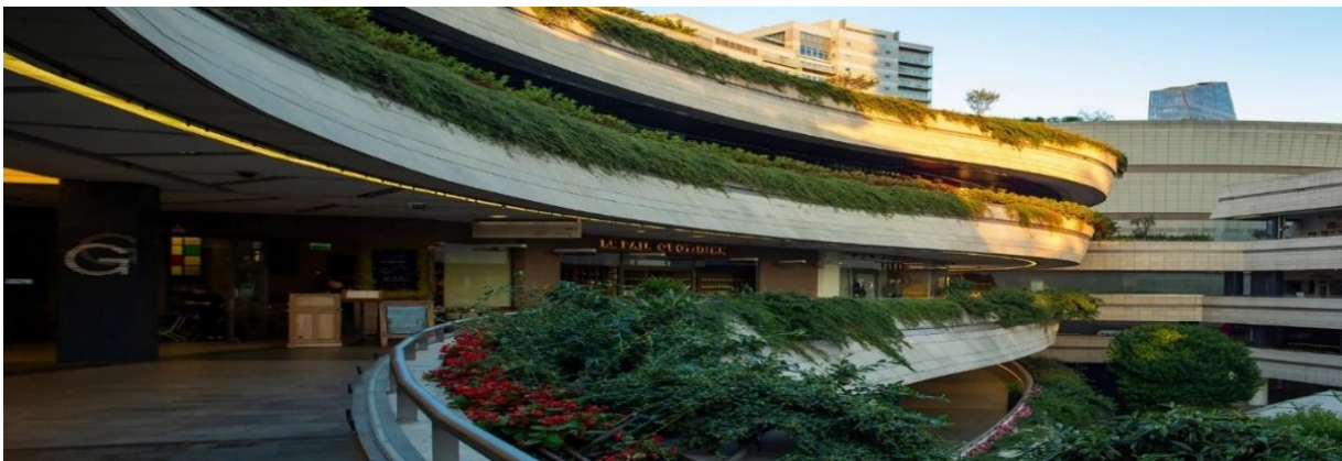
Fig.12. Kanyon Shopping Center Vertical Garden Application Between Floors (URL-12, 2026)
