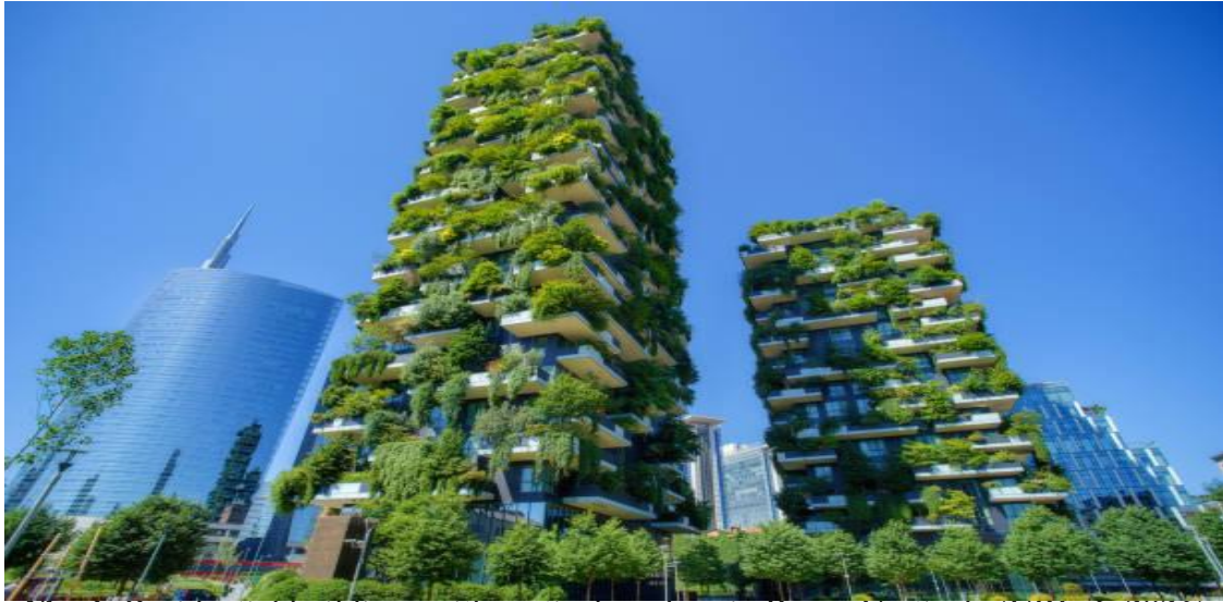
Fig. 6. Residential buildings with vertical gardens in Bosco Verticale (URL-6, 2026)
