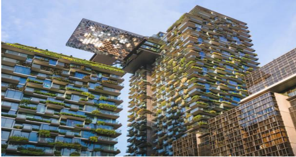
Fig. 7. One Central Park vertical garden application on building facades (URL-7, 2026) 6.1.4. Oasia Hotel Downtown (Singapore)
