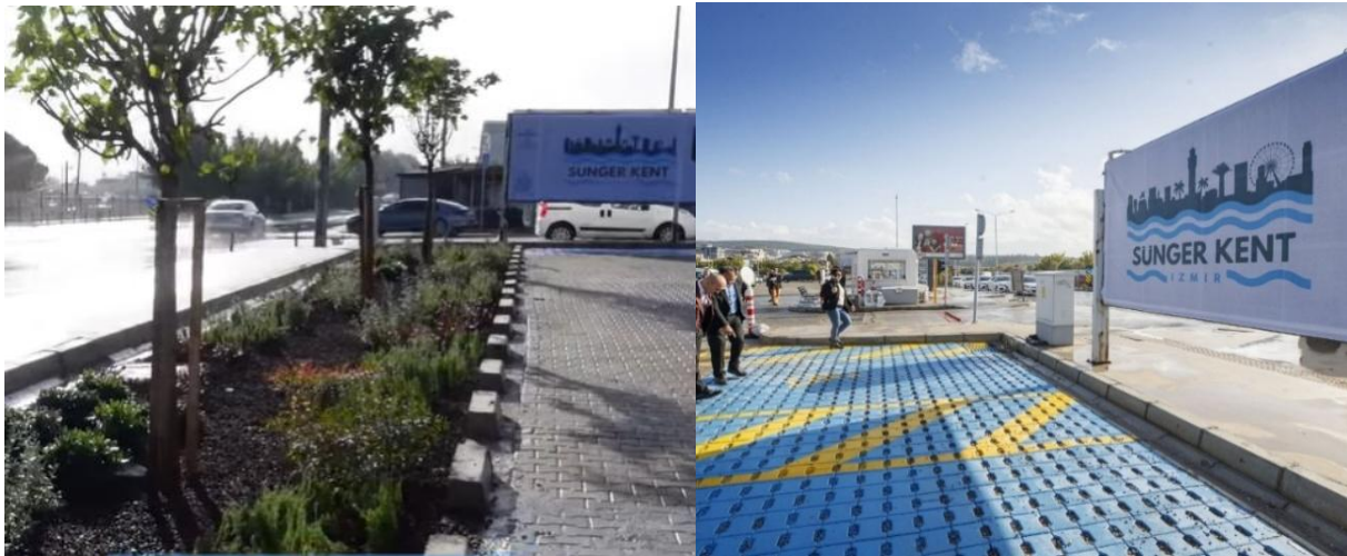
Fig. 14. Sakarya Sponge Parking Lot Permeable Pavement and Rain Gardens (URL-14, 2026)
