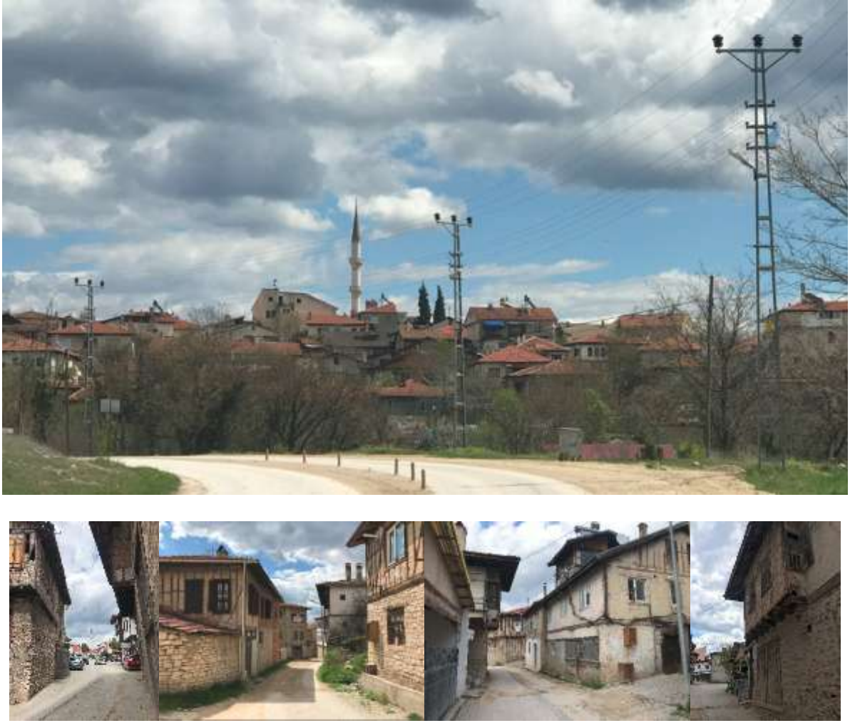
Fig. 2. General view of the architectural heritage of Karabük, Safranbolu, Yazıköy.
