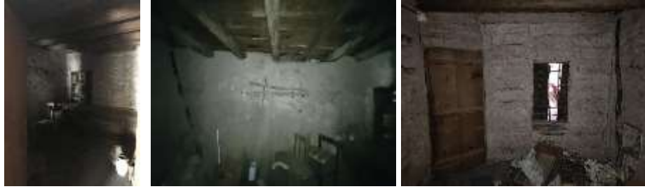
Fig. 9. Mid-Floor Room 2 Space
