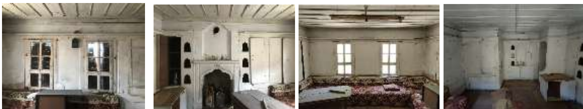
Fig. 8. Mid-Floor Room 1 Space
