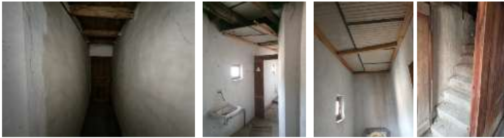
Fig. 12. View of the Staircase with Toilet and Aralık
