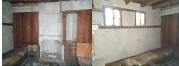
Fig. 16. View from Upper Floor Room 4
