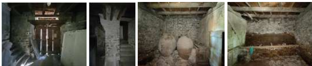
Fig. 6. View of the ground floor stony area, warehouse (old cellar) and cellar.
