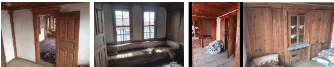
Fig. 14. View from Upper Floor Room 2
