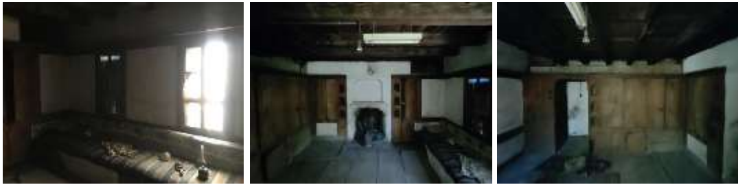
Fig.10. Mid-Floor Room 3 Space
